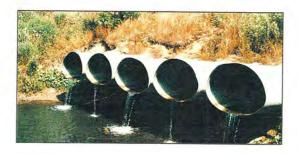
Figure 10. Above.Culverts on Amberlea Creek close to West Shore Community Centre (left) and on Pine Creek at Douglas Park (right). These are responsible for enhanced erosion and lowering of the creek bed and the production of sediment that is transported to Frenchman's Bay (Fig. 16).
