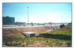
Figure 9. Culvert on Pine Creek where it passes under Highway 401. Note erosion of embankment and that water and sediment from the highway is free to drain to creek (see Fig. 16).
